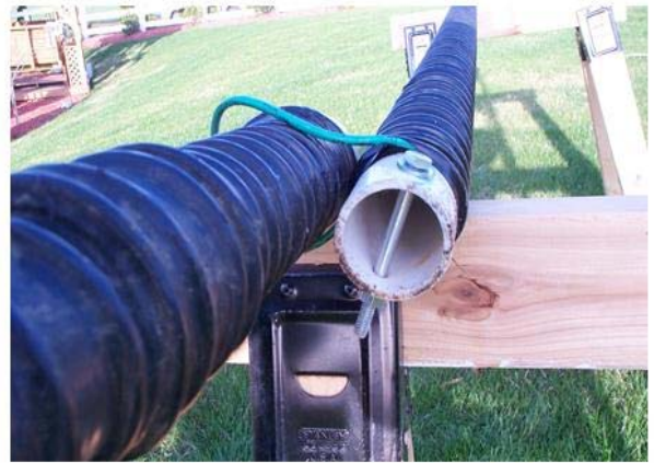
The bolted union between the lower 10' sections.
