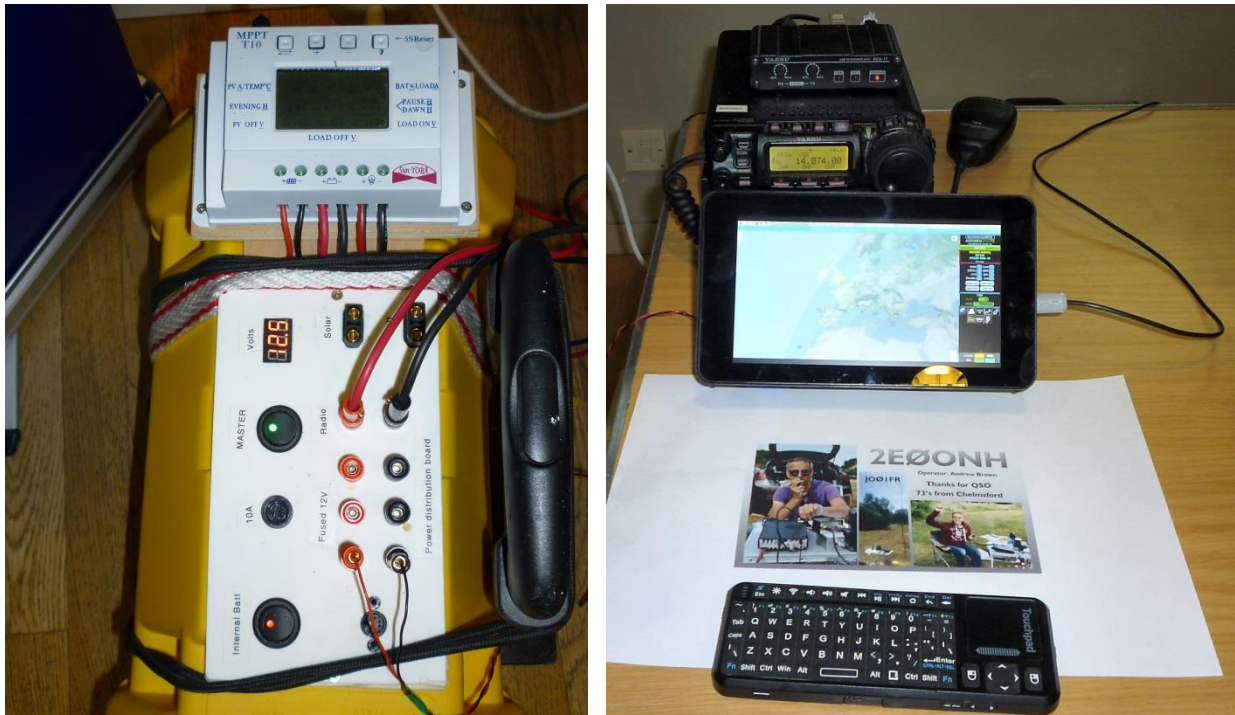
Andrew 2E0ONH: Power supply and Raspberry Pi with Yaesu FT-857 and SCU-17 USB Interface unit
