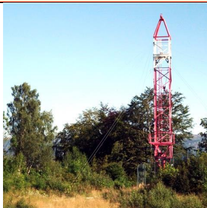
Today – a few restored sections 24m high – used for the LA1ASK HF antennas
